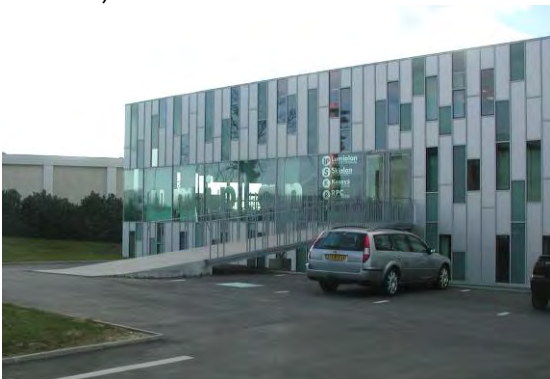
Percements non standards / Alternance vitrage-bardage
